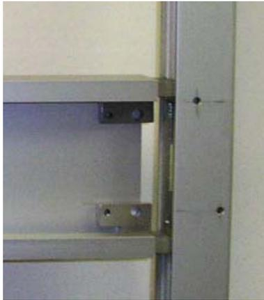
With the door stiles loose or unassembled, insert the MP010M Muntin Channel between the stiles and over the mounting clips. Then finish door assembly and tighten.
