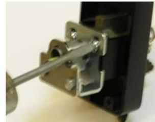
Mount MP021 Cylinder Mounting Assembly to active stile using two 1/4-20 x 2" PHMS.
